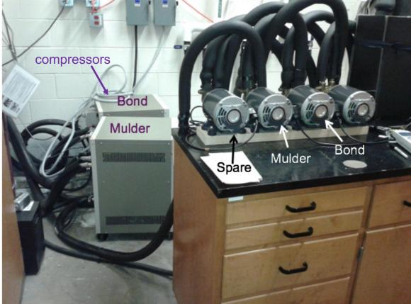
The pumps pump water from one common reservoir into the three separate compressors and then into a heat exchanger. The pumps are cleverly plumbed together so that the spare pump can be used for any of the three compressors:
