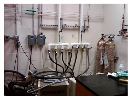
The temperature of the building chilled water can be monitored from the thermometer attached to the "Chilled Water Supply" pipe in MSB1425 (the room right next to Mulder).
